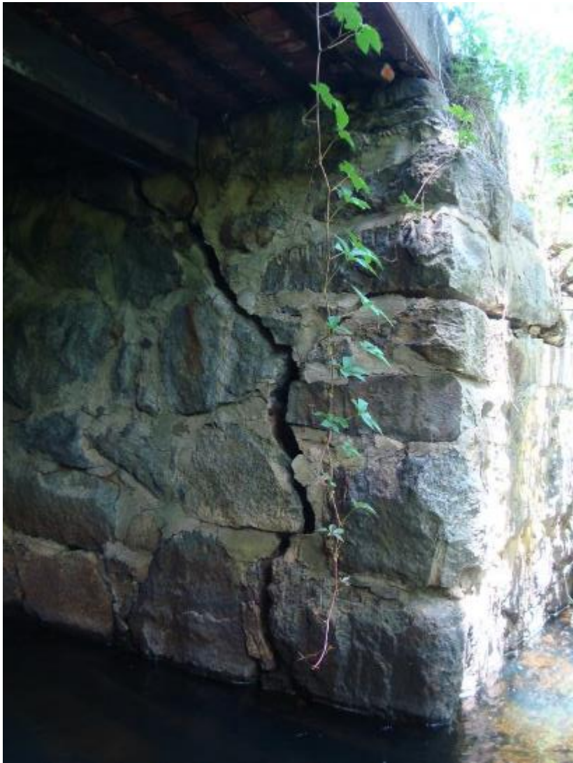
View of South end – Note large crack in stone masonry
