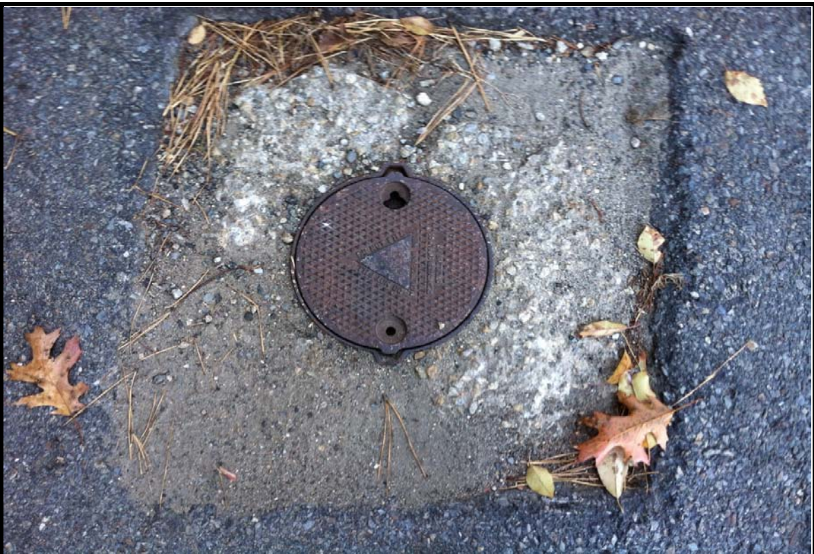
Description - Condition of Monitoring Well Road Boxes on Sculley Road
