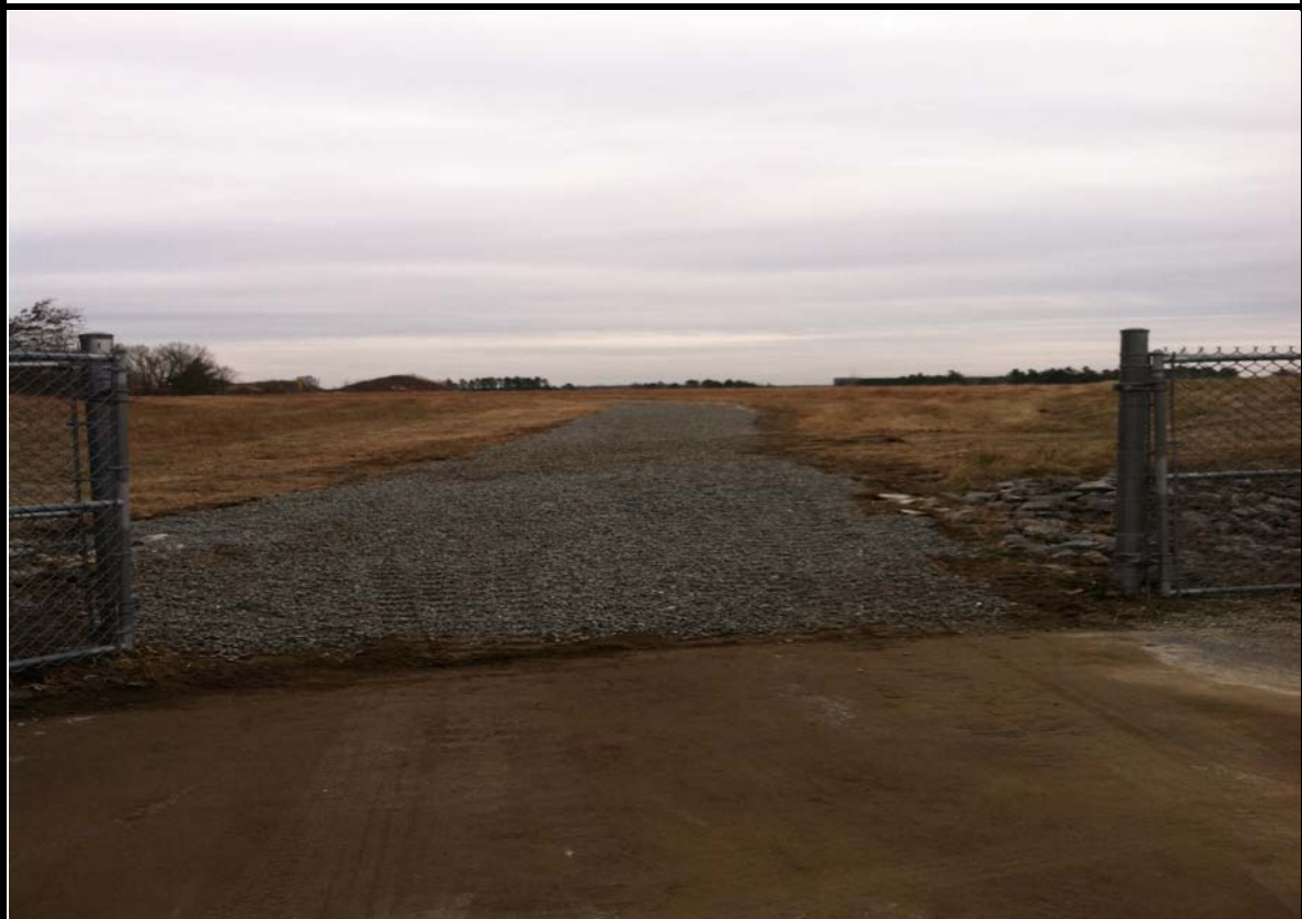
Description - Northern Access Road Repaired
