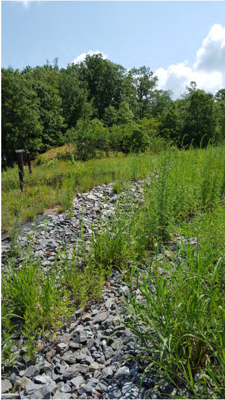
Riprap at barrier wall
