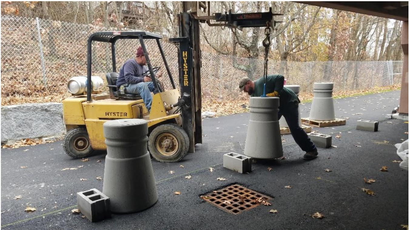
Parking Bollard installation
