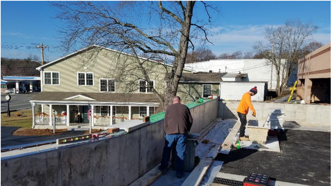
Wall Cap installation
