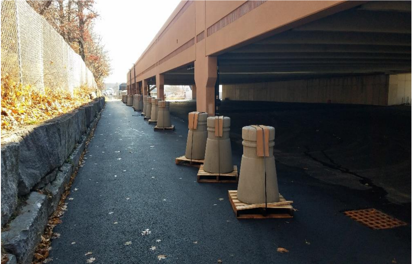
Parking Bollard Installation
