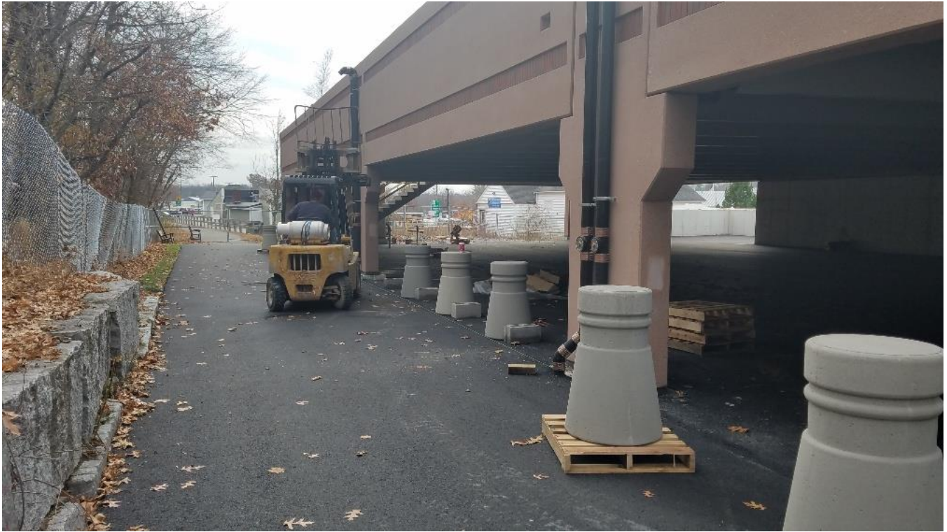
Parking Bollard installation
