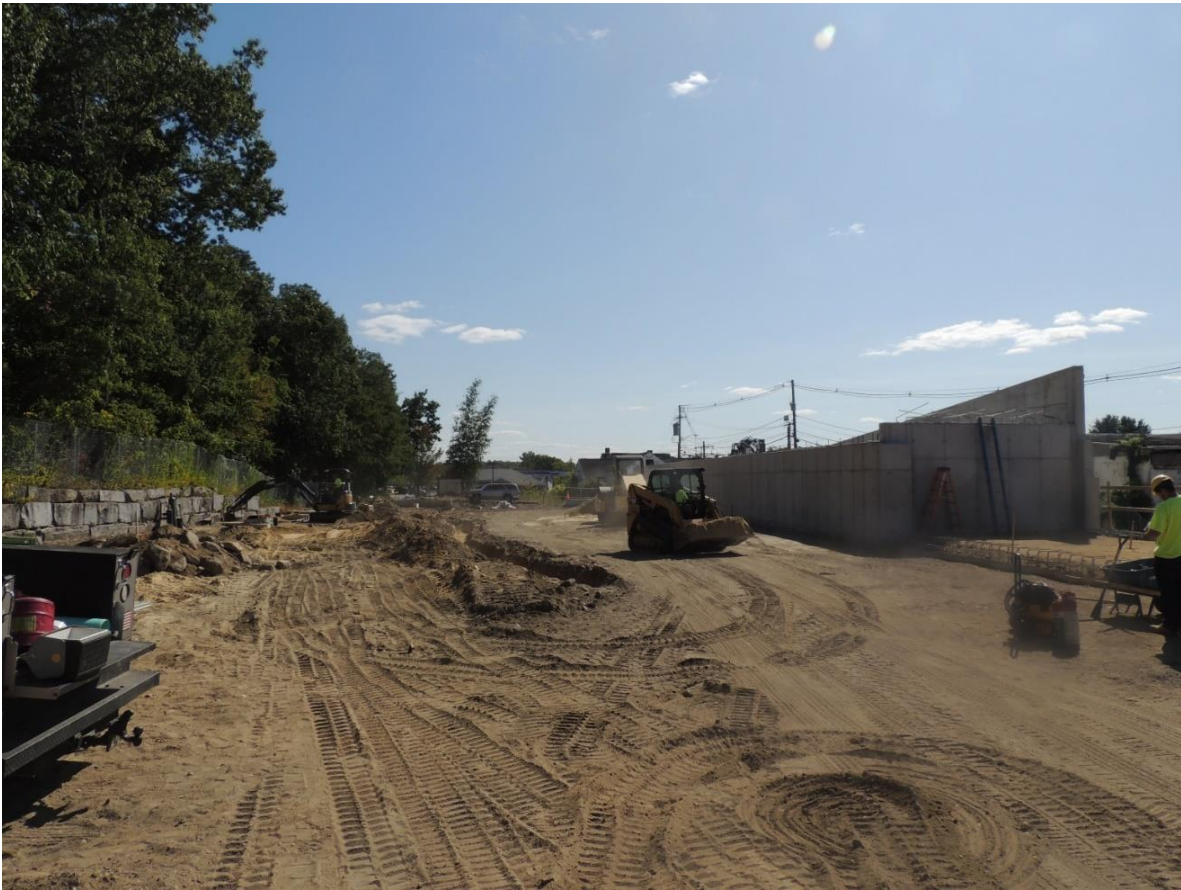
Site Backfill Compacted
