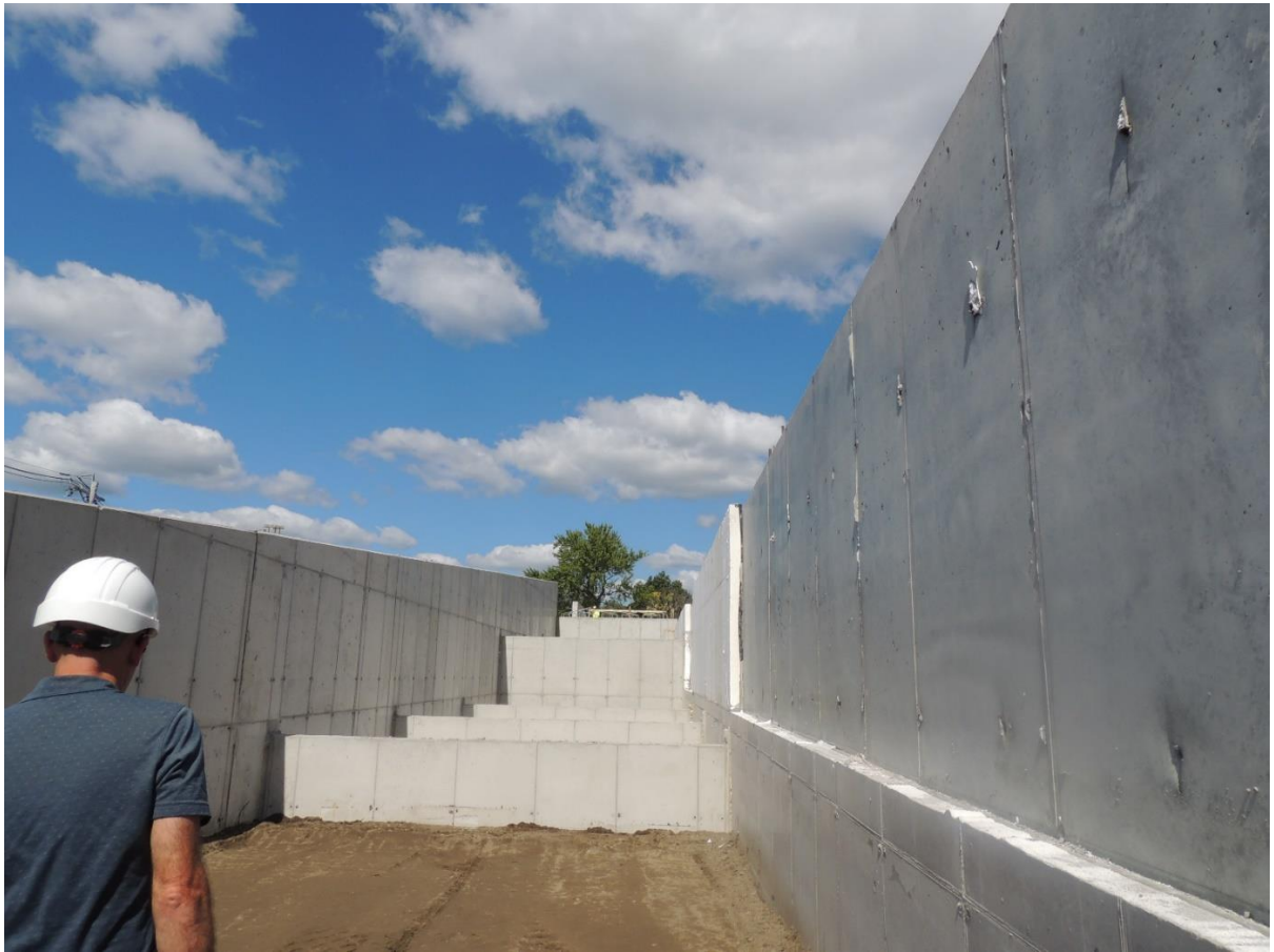
South Ramp Backfill Foundation Compacted
