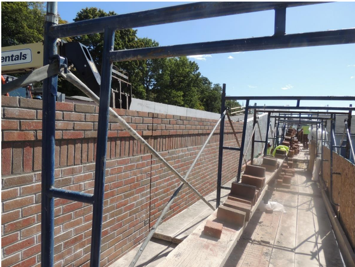
Masonry Brick Being Placed
