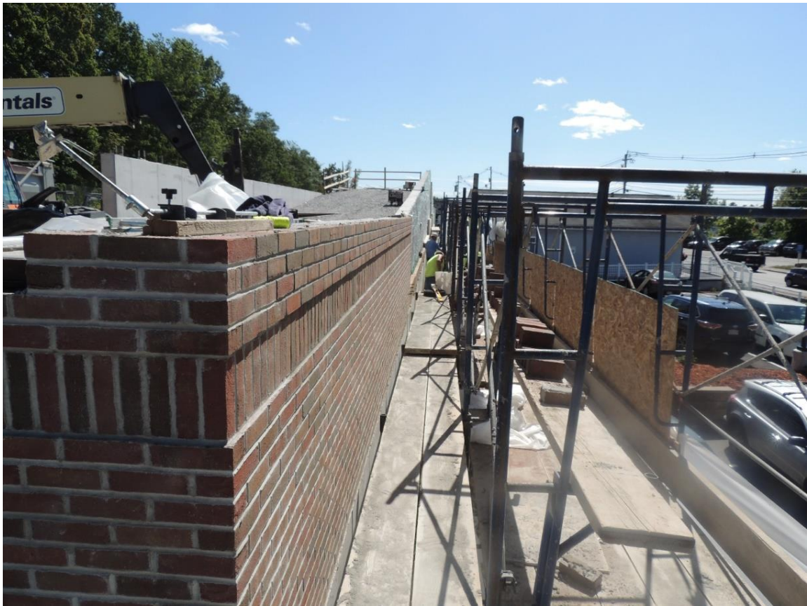
Masonry Brick Being Placed
