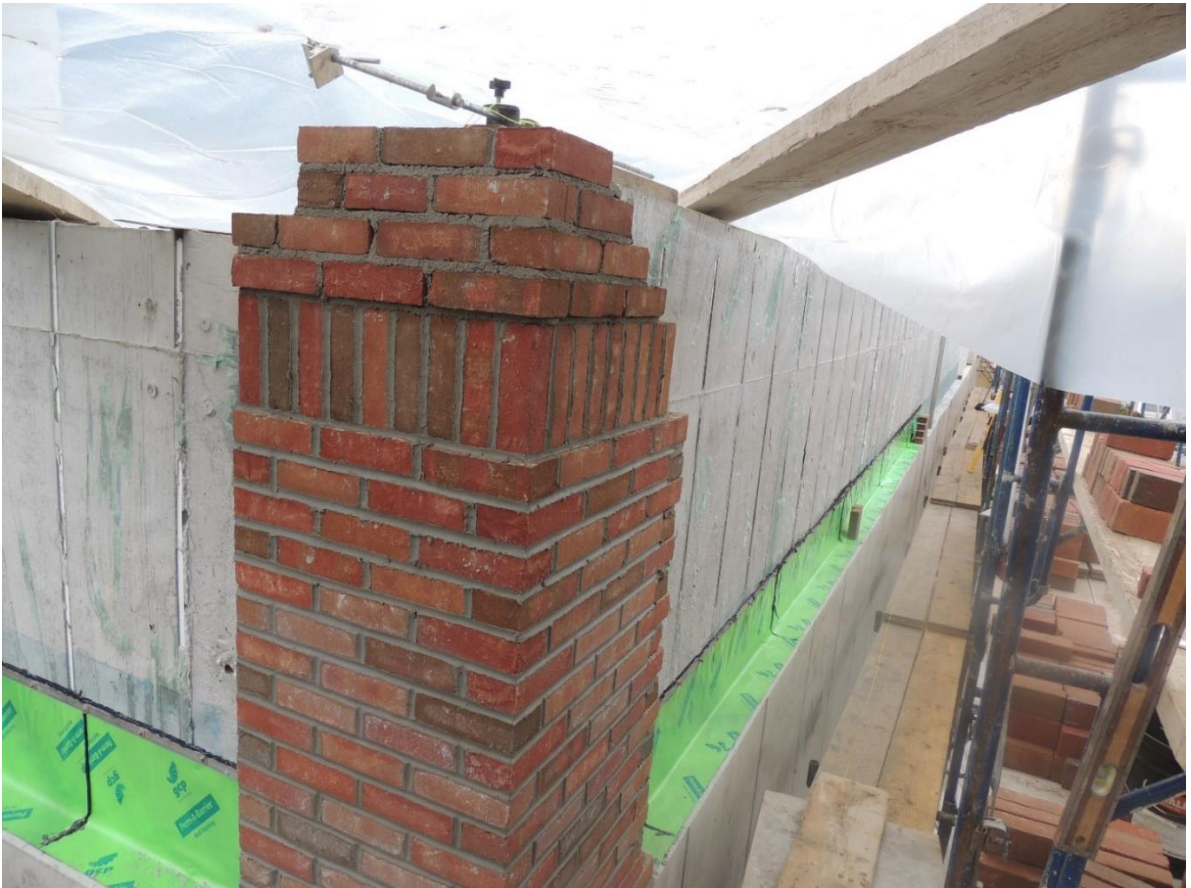
Masonry Brick Being Placed
