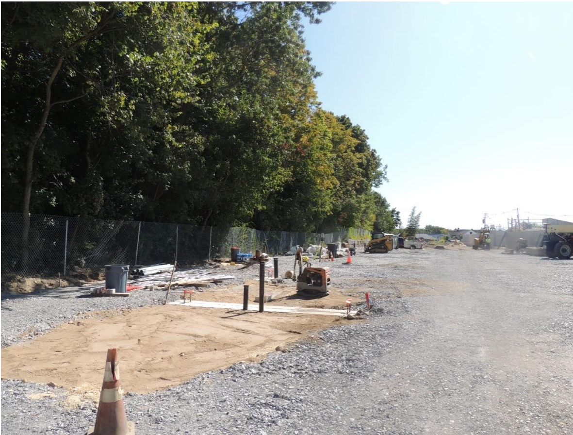
Rail Trail Gravel Sub-Base Compacted
