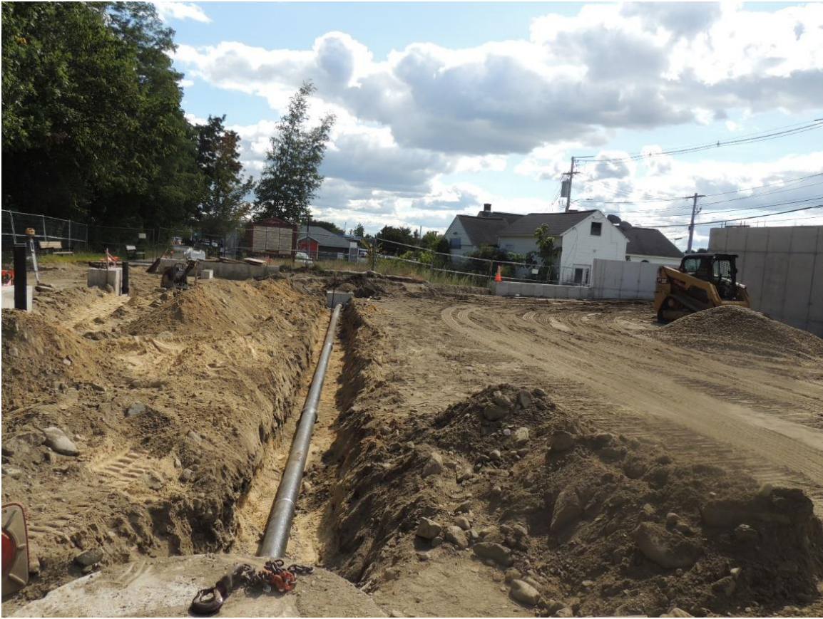
Site Under-Ground Drainage
