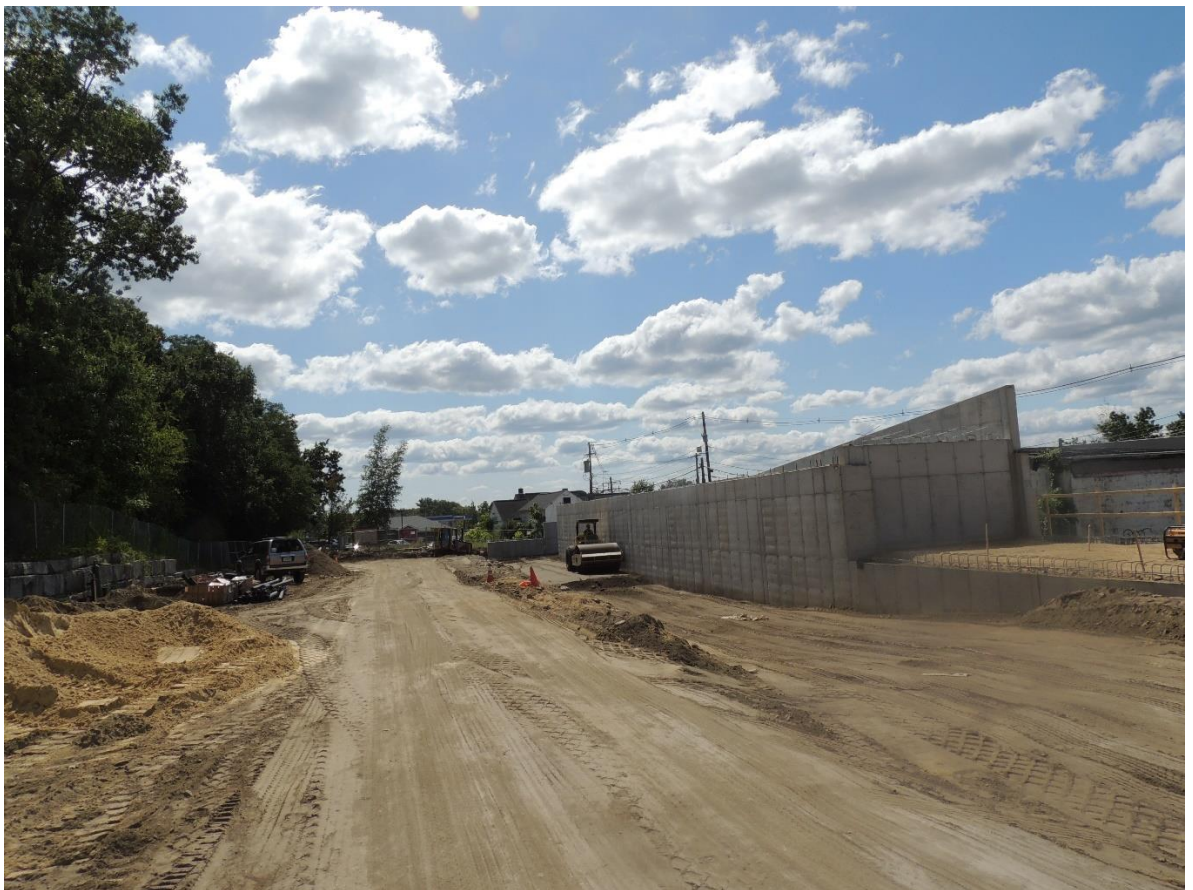
Site Backfill Compacted
