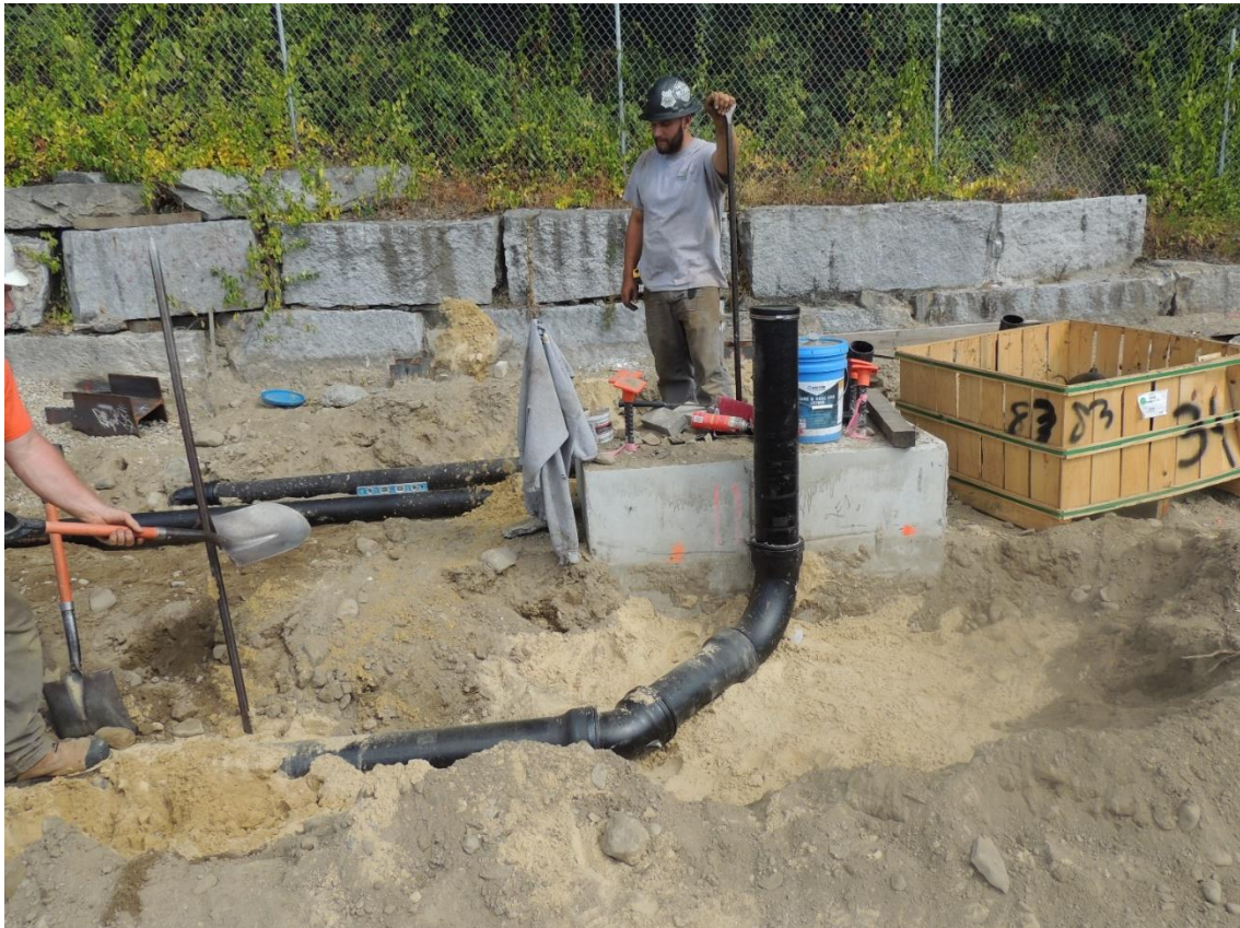
Vents, Drain Lines Piping Being Set
