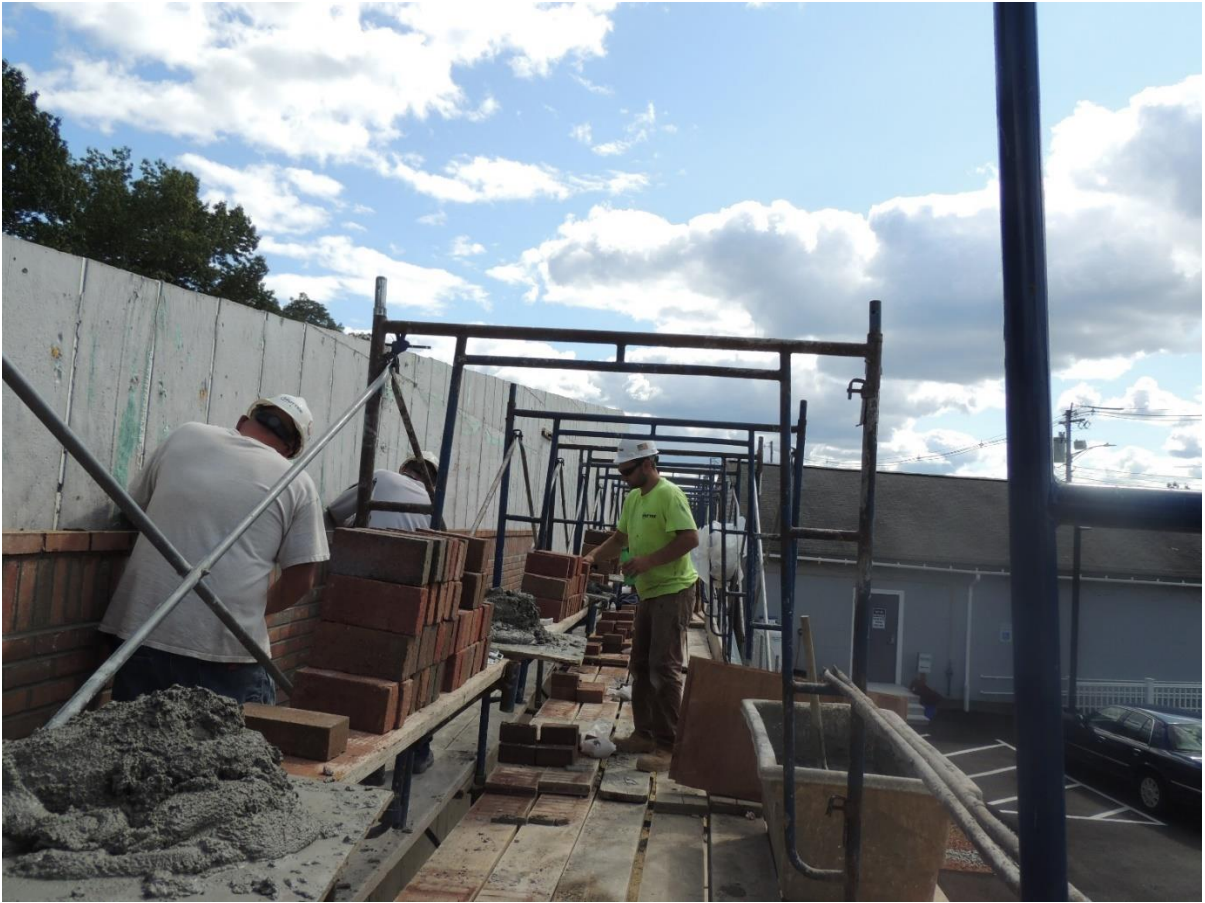
Masonry Brick Being Placed
