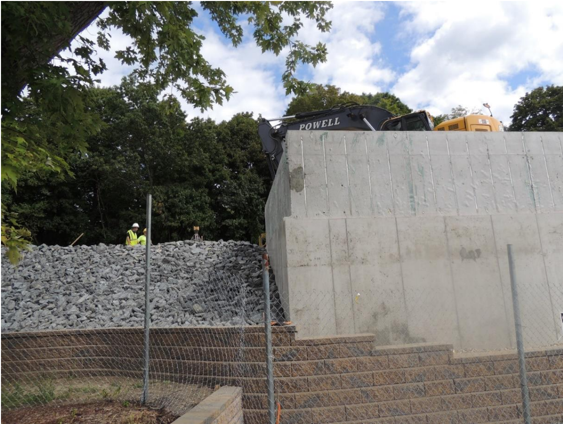
Rip-Rap for Slope Stabilization Installed at Northwest
