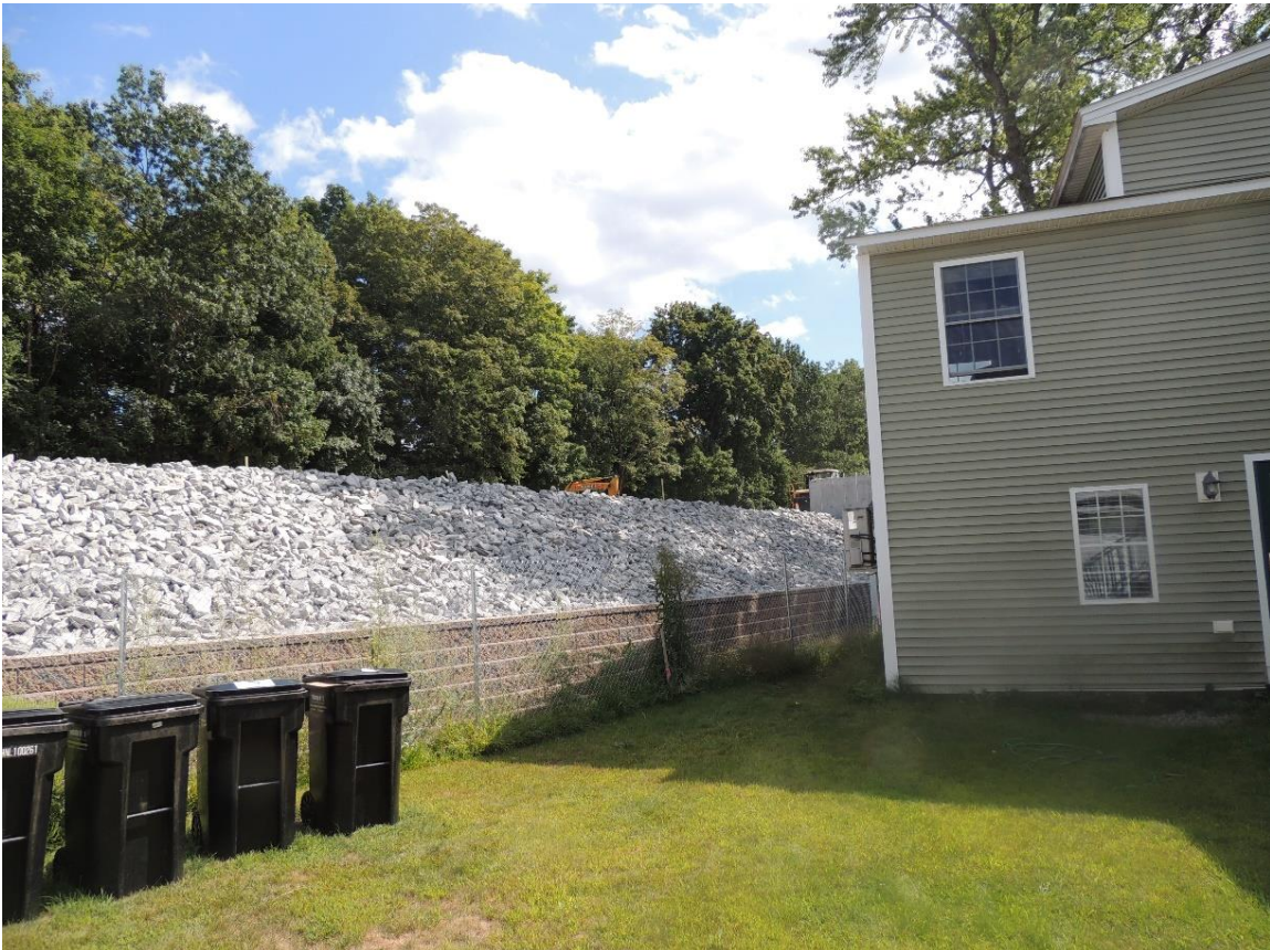
Rip-Rap and retaining Wall Completed at Northwest
