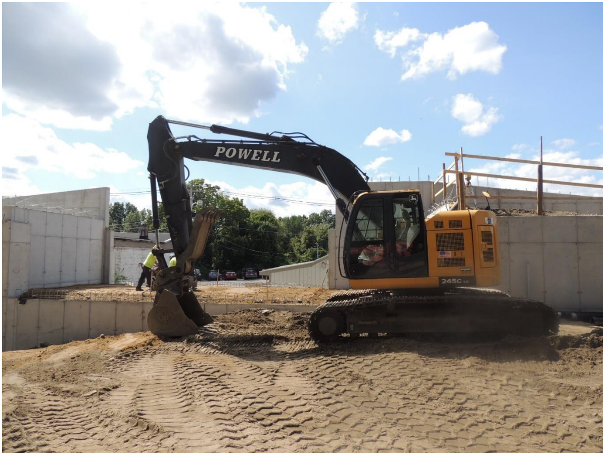
Site Backfill Compacted
