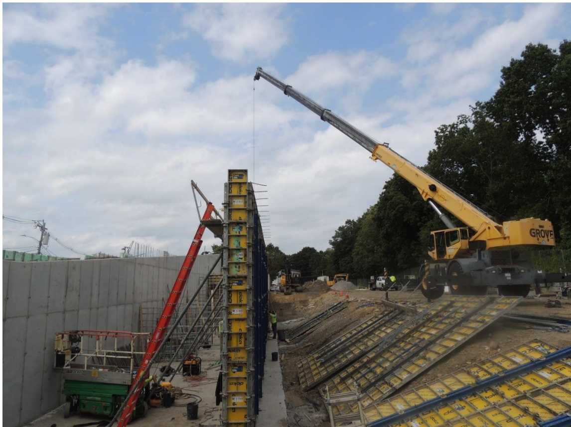
South Ramp Foundation Forms
