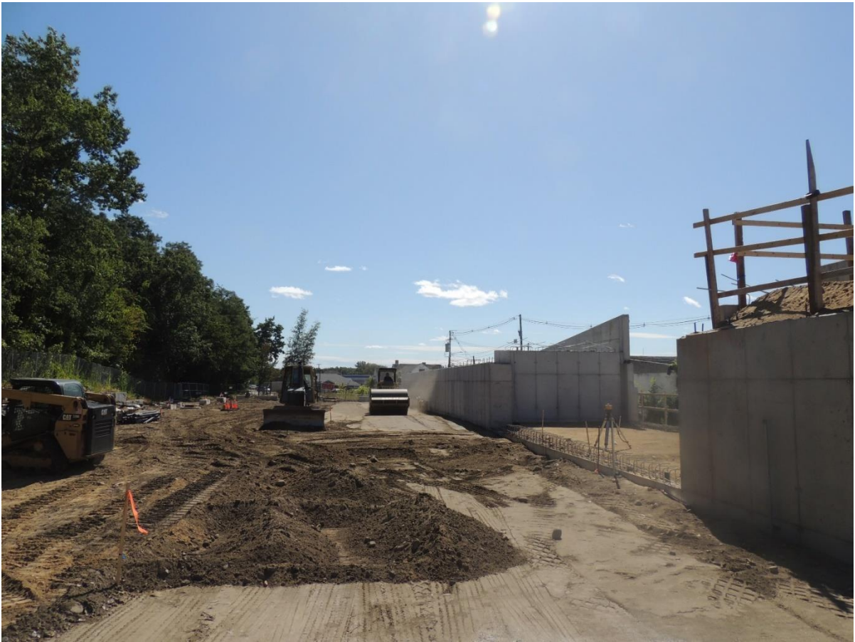
Site Backfill Compacted
