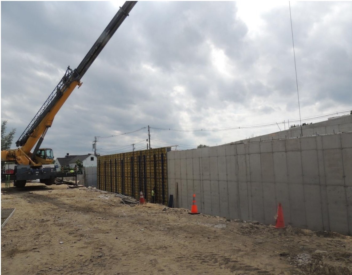
South Ramp Foundation Forms
