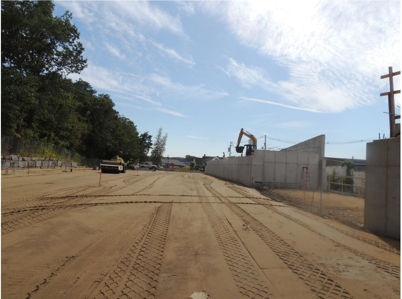
General Parking Area Backfill compacted
