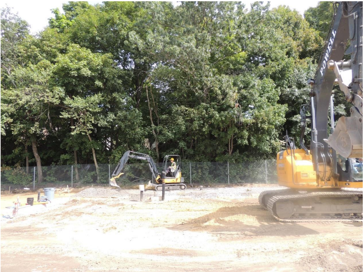
Rail Trail Gravel Sub-Base Compacted
