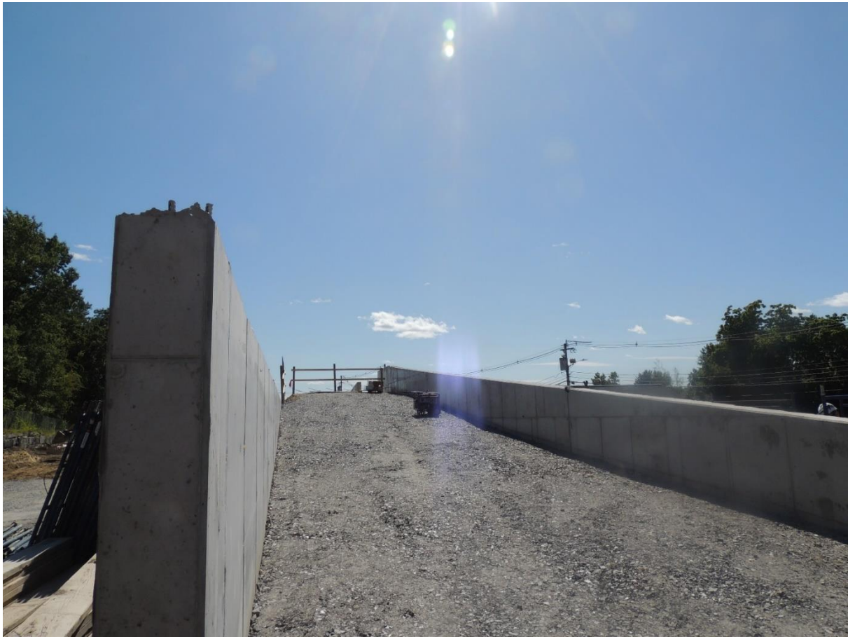
Ramp Gravel Sub-Base Compacted
