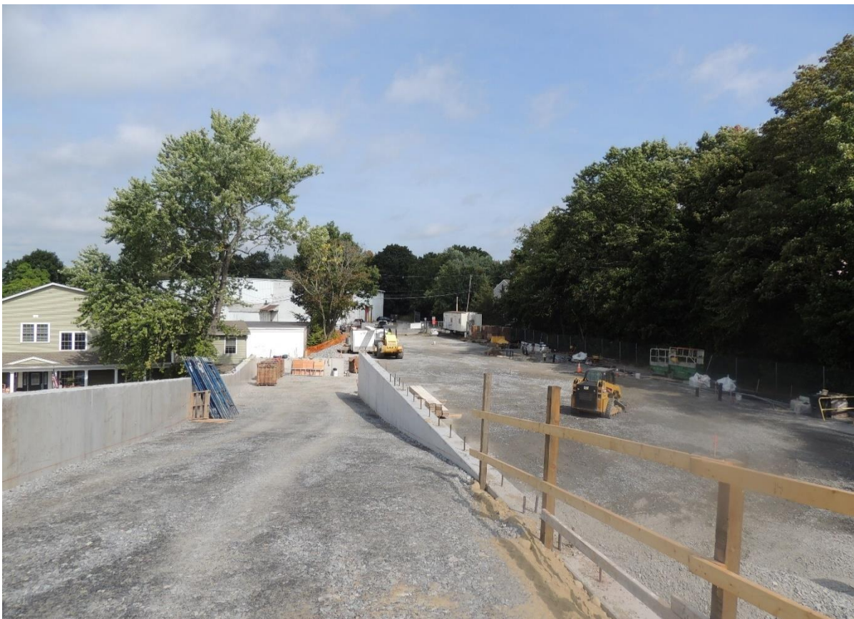
Ramp Gravel Sub-Base Compacted
