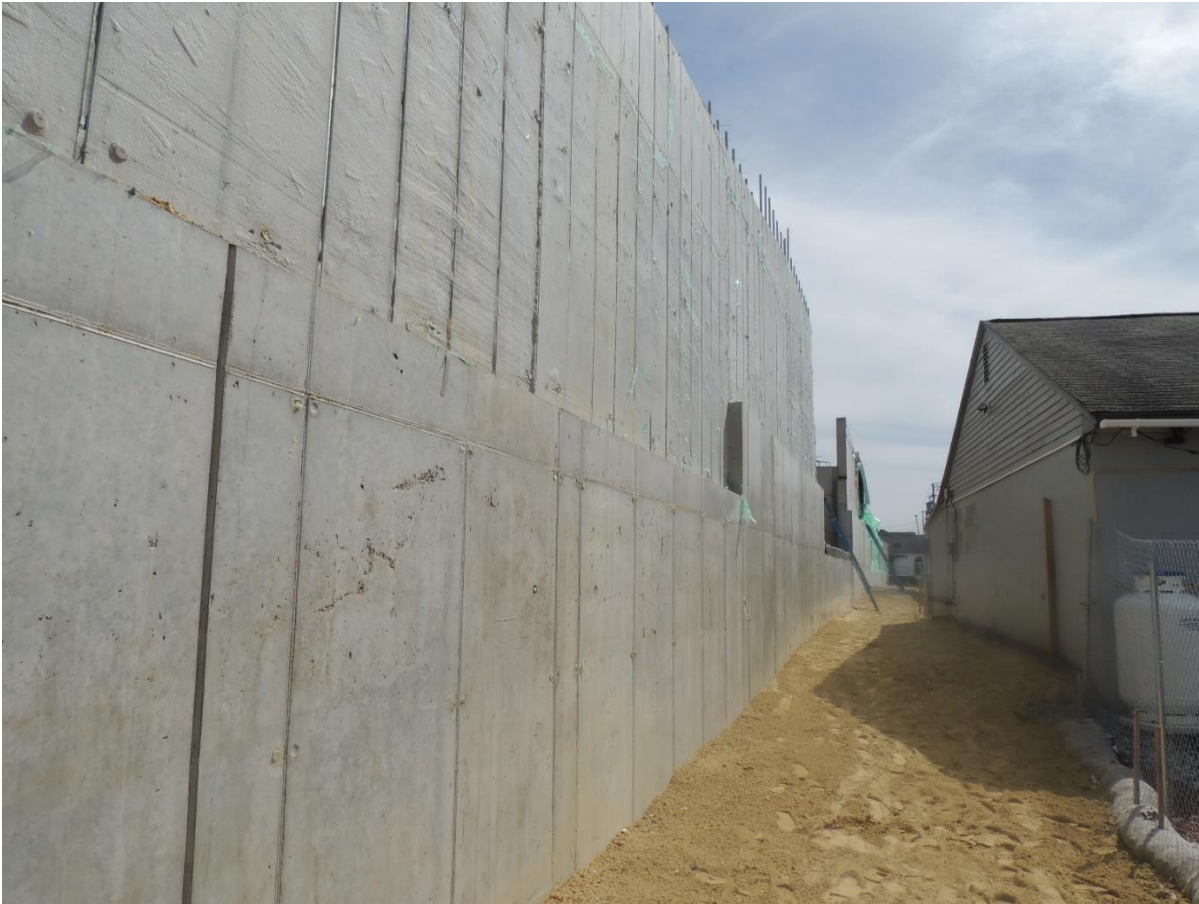
Backfill Foundation Compacted
