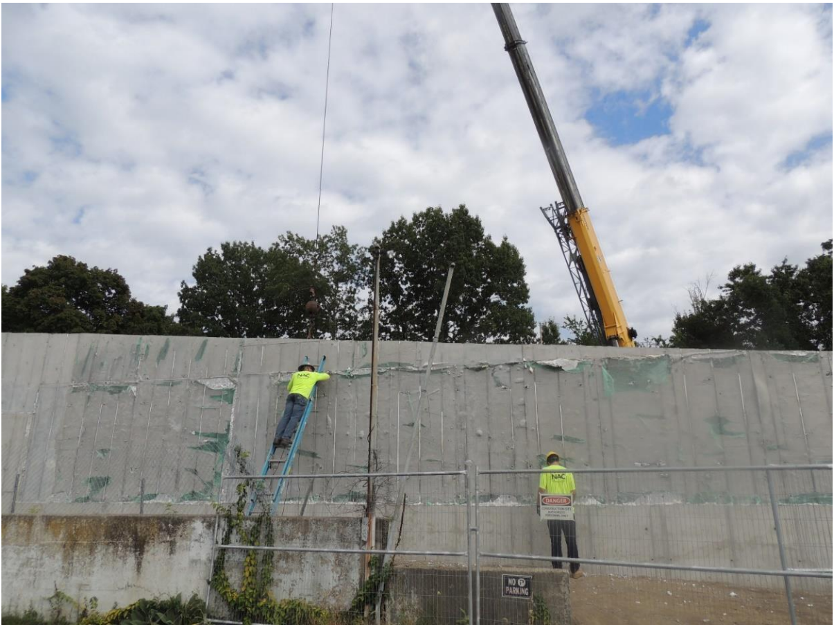
Block-out Foam Being Removed
