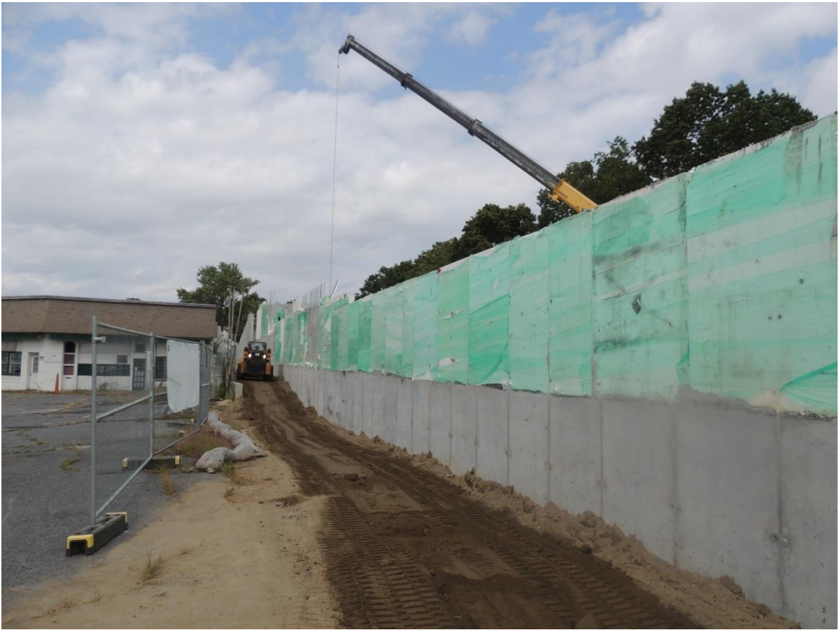
Backfill Foundation Compacted
