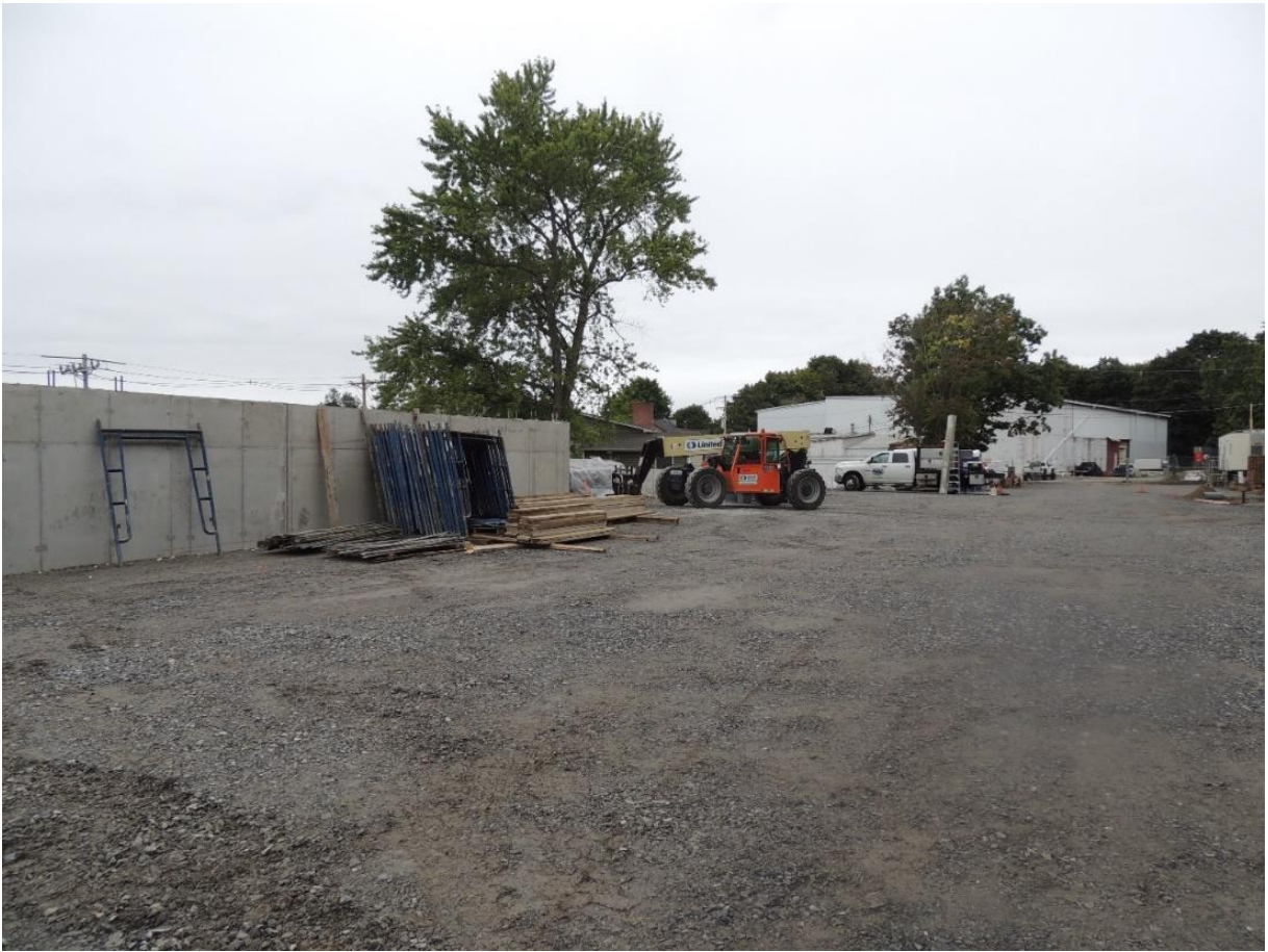
Parking Lot Gravel Sub-Base Compacted
