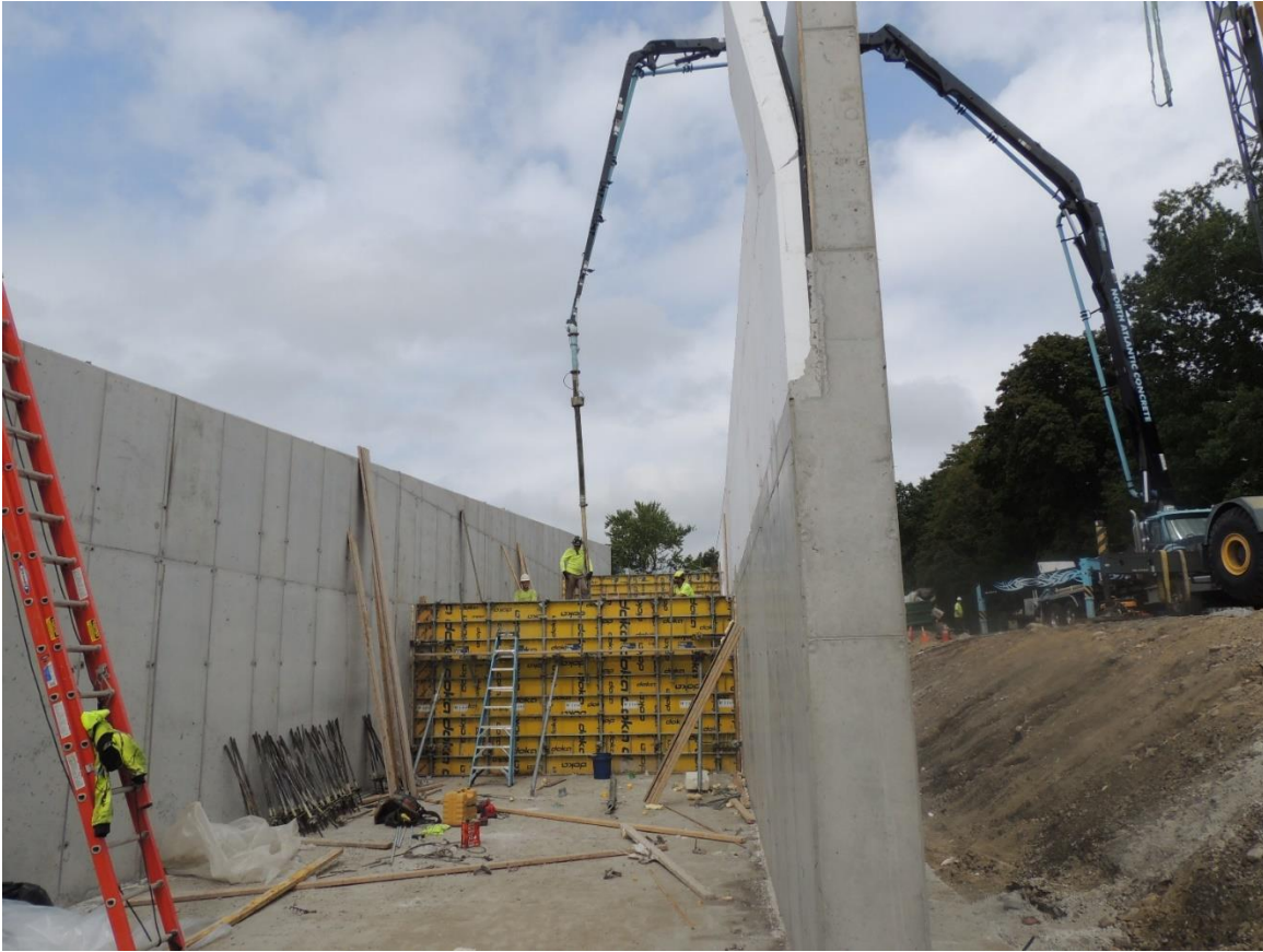
Intermediate Walls Foundation (Concrete Pump Beyond)
