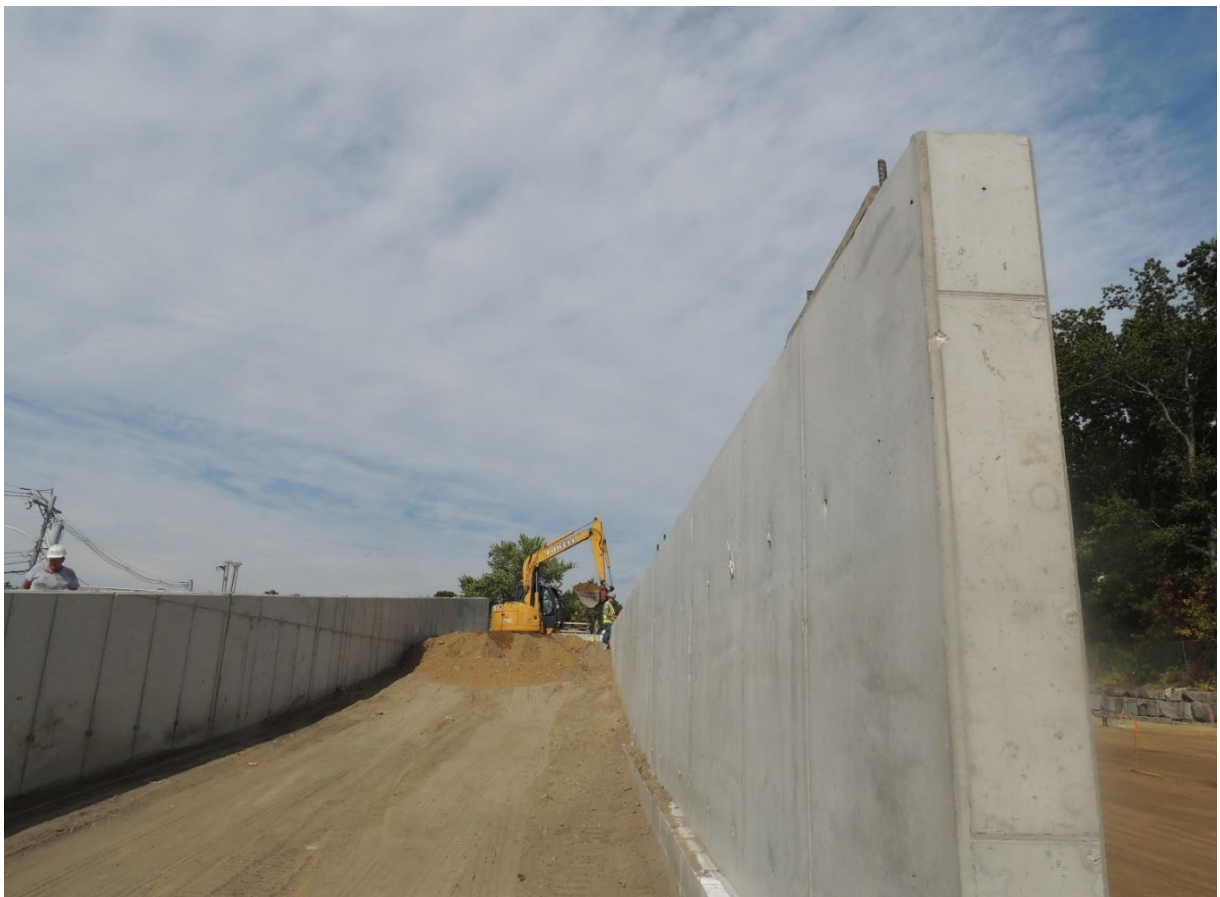
South Ramp Backfill Foundation Compacted
