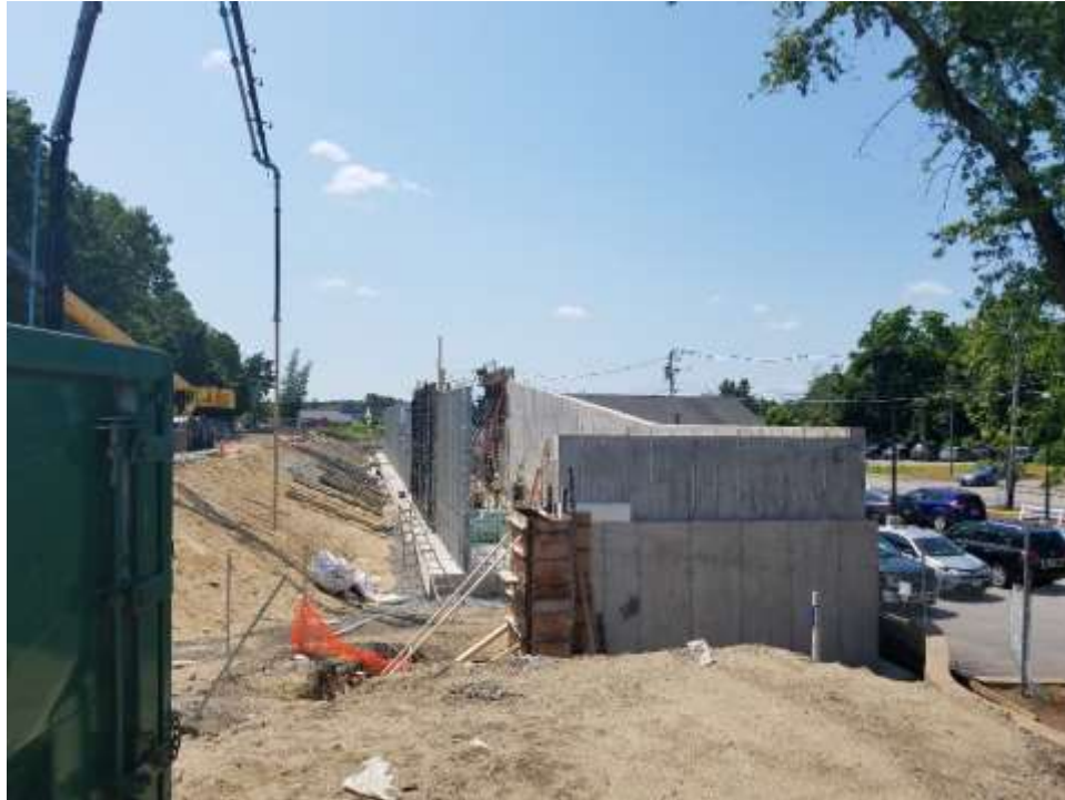
Ramps Retaining Wall Foundations
