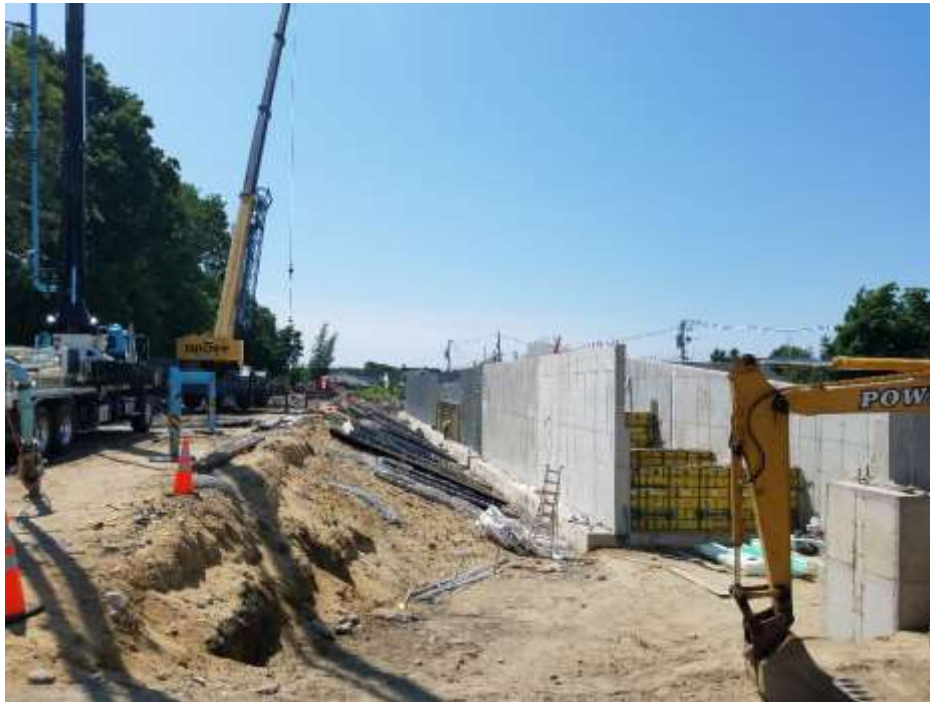
Ramps Retaining Wall Foundations
