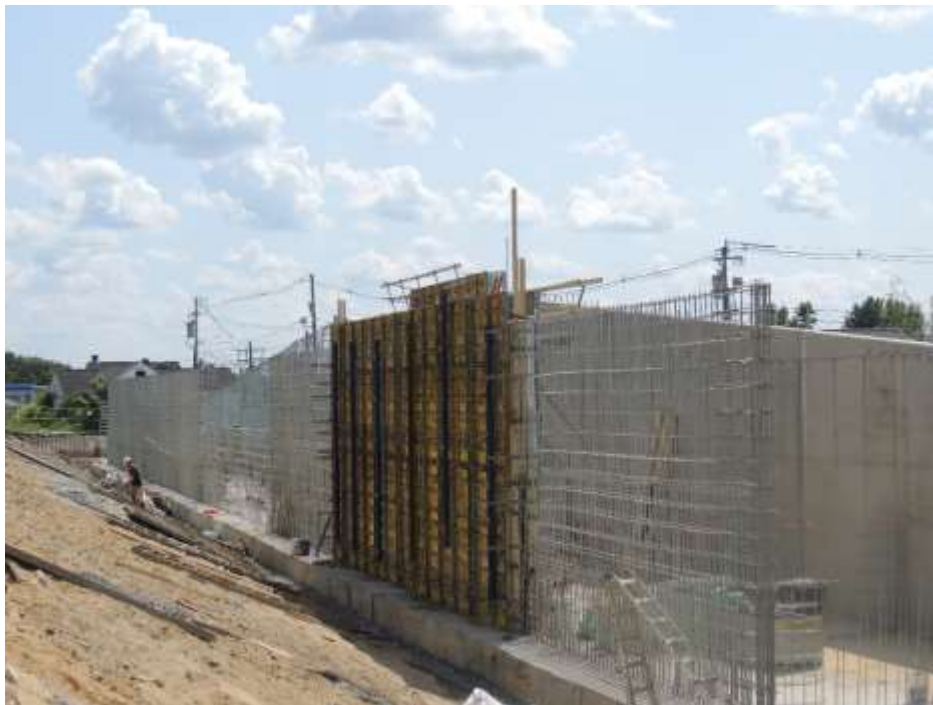
Re-Bar Retaining Wall Foundations
