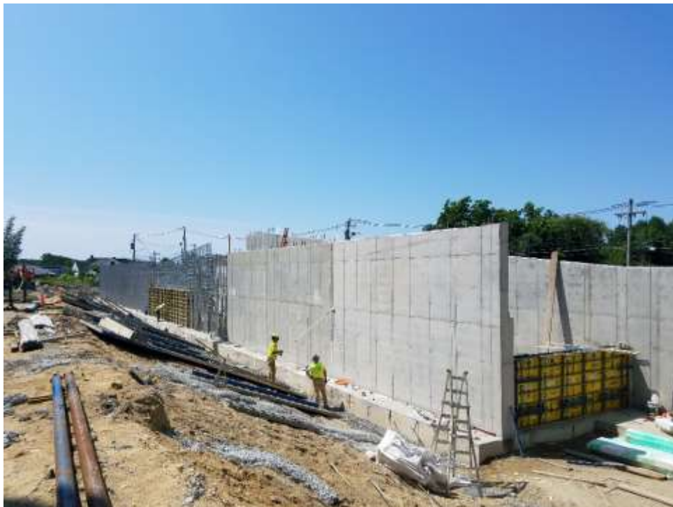
Ramps Retaining Wall Foundations
