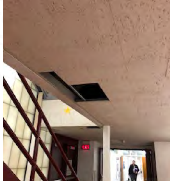
Missing panels in hallway ceiling
