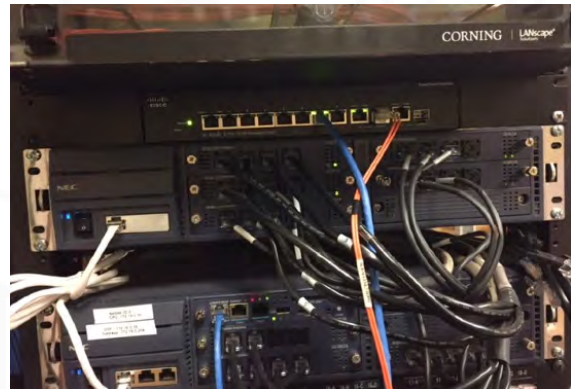
NEC phone system in MDF rack
