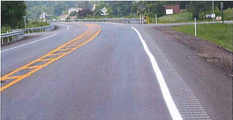
Example of flush divisional island constructed with painting and rumble strip scoring. Alternatively, the island could be constructed of concrete.
