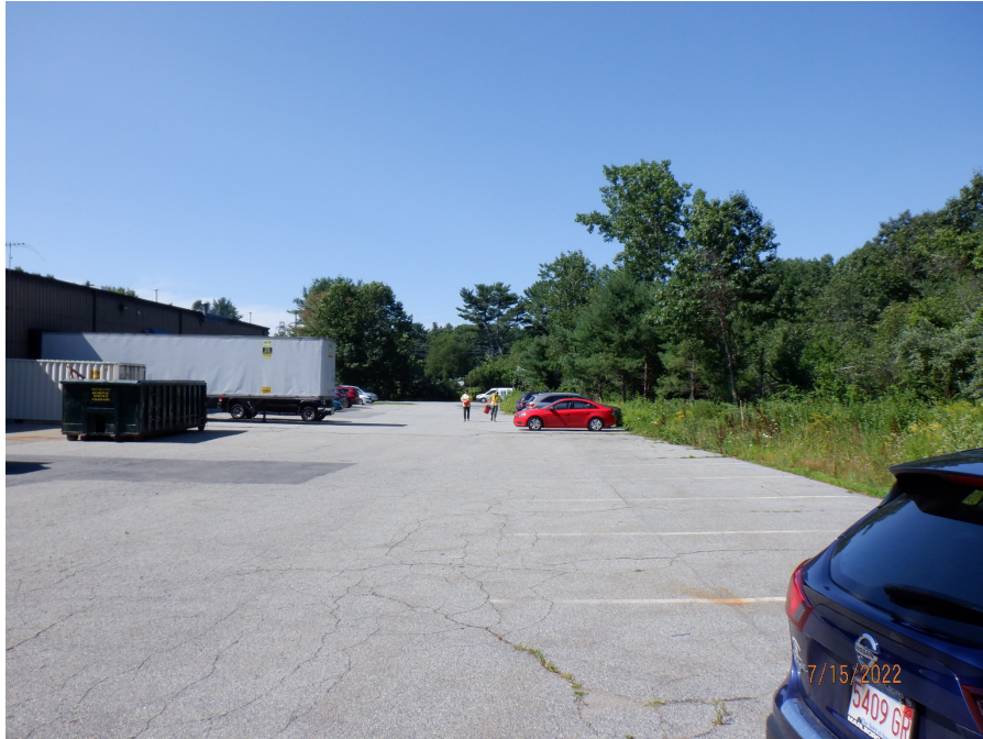
Photograph 1: Existing building on the site, taken from the rear parking lot.
