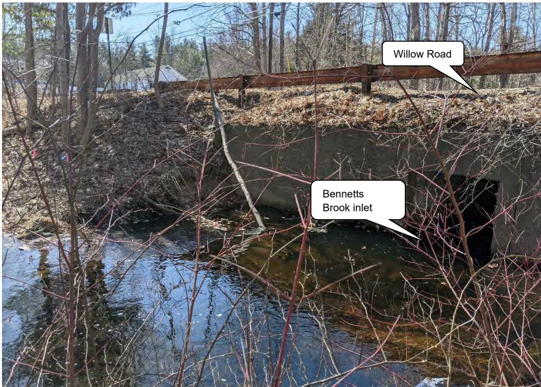
Photo 06 –View east at the Bennetts Brook Inlet
