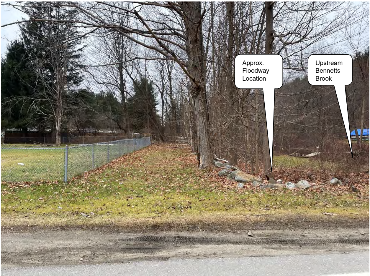
Photo 2 – Upstream Side of Culvert at Bennetts Brook
