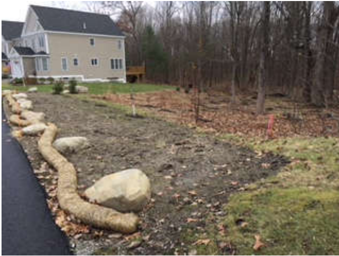
Area #1: stoned shoulder was restored with loam and seed
