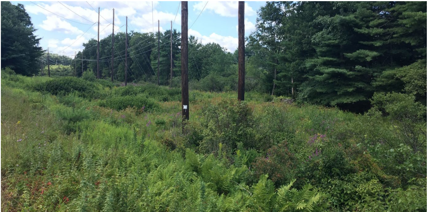
Photo #2: View of emergent wetland AY-W18, looking towards Structures 9/10. No permanent impacts to BVW are proposed. Activities within BVW include in-kind structure replacement (no change in structure footprint), and temporary matting for access and work pads. Facing southwest.
