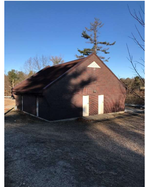
Central Avenue Pump Station
