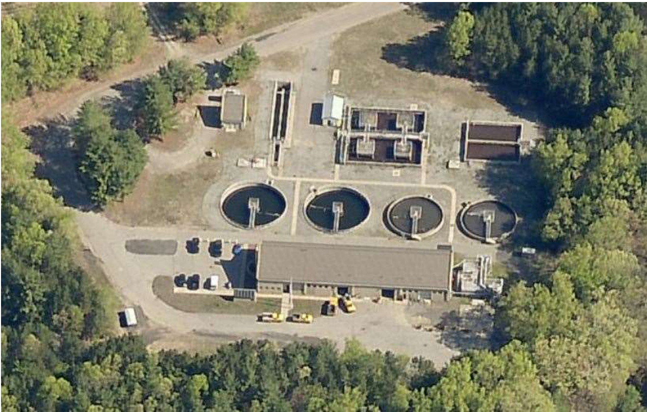
WWTP Year Built 1982
