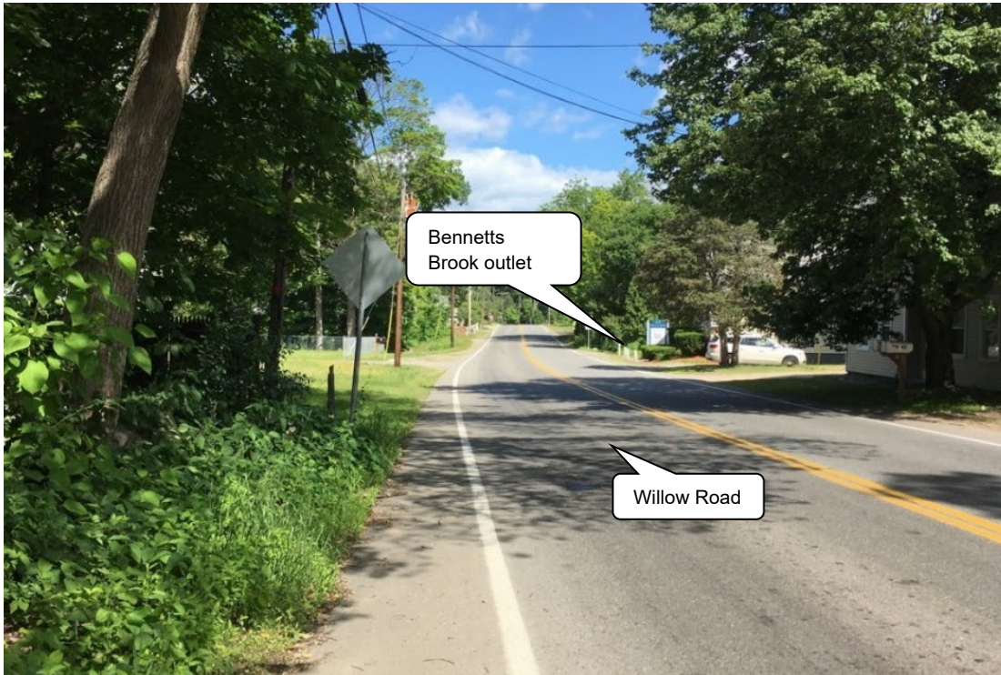
Photo 03 – Approx. Sta. 18+00, View northwest down Willow Road towards Bennetts Brook crossing
