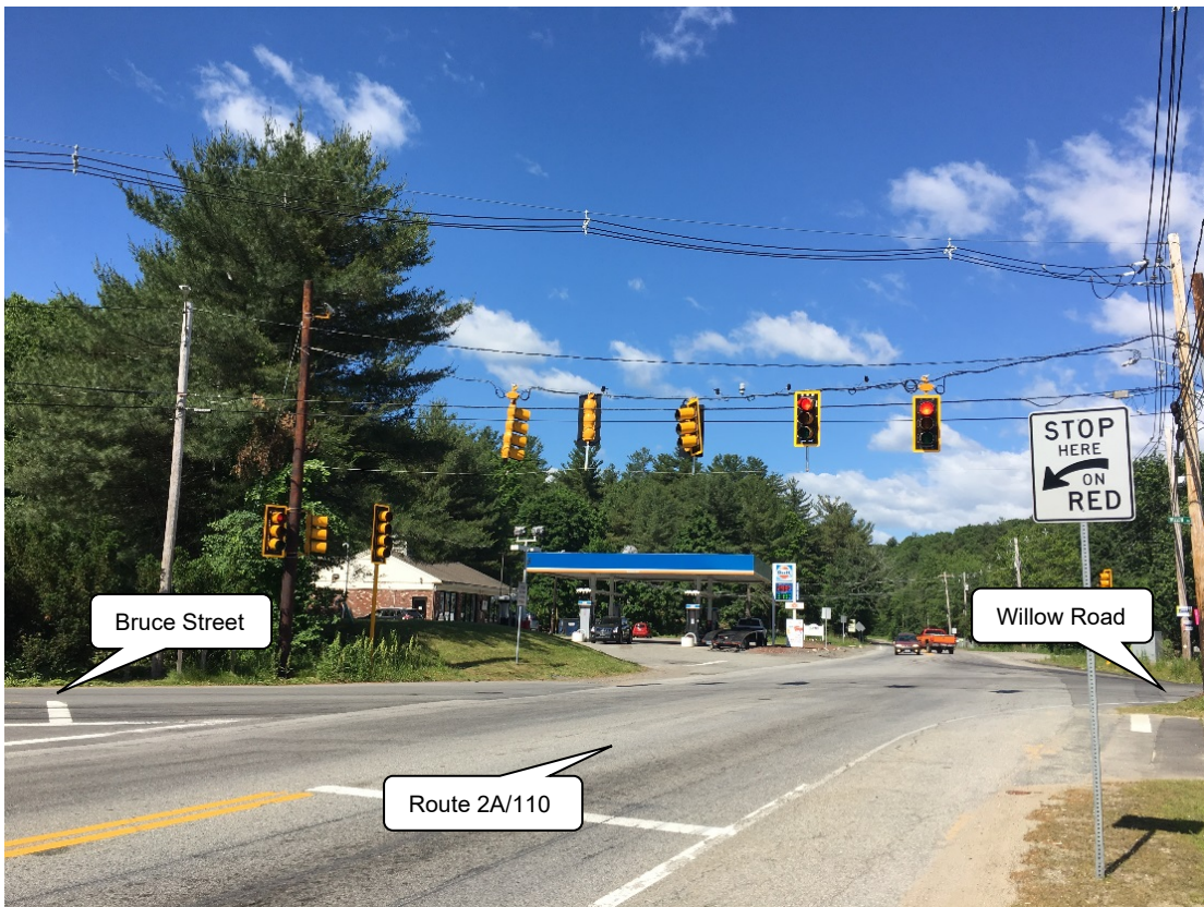
Photo 01 – Approx. Sta. 8+00, View West on Route 2A from westbound stop line at the intersection
