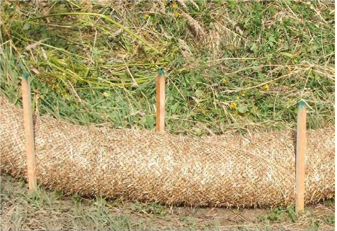
STRAW WATTLE – SHALLOW SLOPE ( \leq 4:1 ) (ALTERNATE STAKING)
