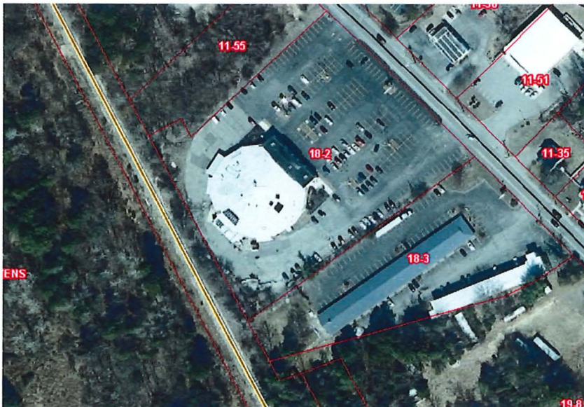
22 Fitchburg Road (Lot 18-2) with supermarket, above
