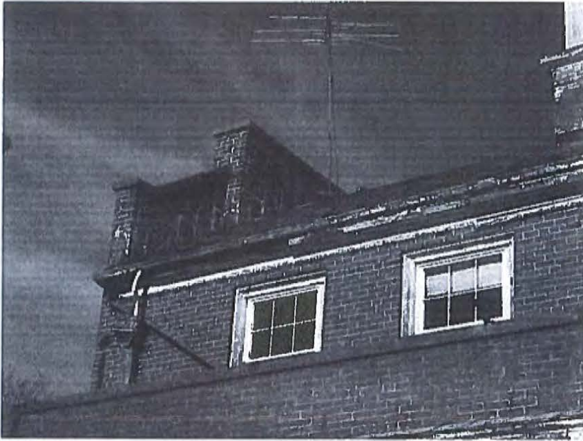
(3.) 1934 Upper Stepped-Brick Gable (South Elevation/Inner-Face)
