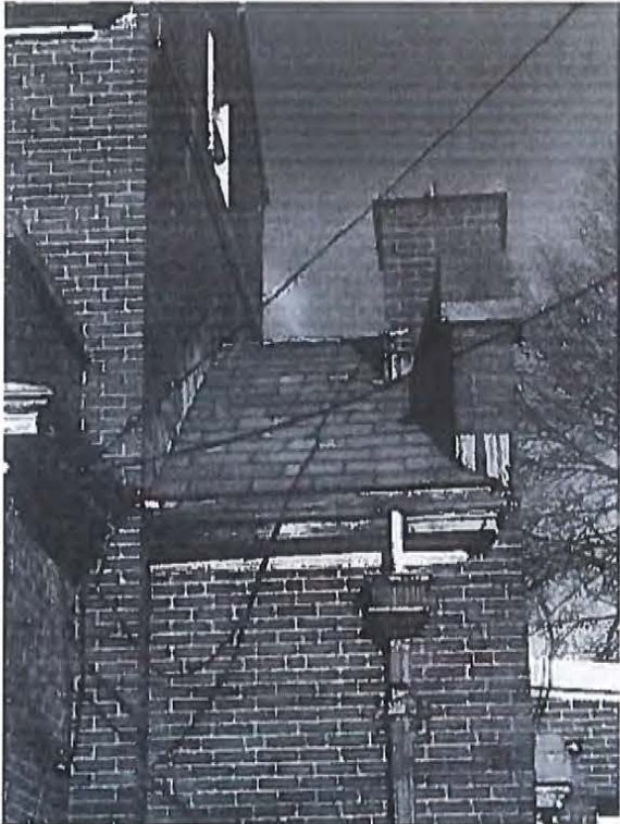
(9.) 1934 Slate Roof – Lower (North-Side/East Elevation/Portion Visible from Washington Street)
