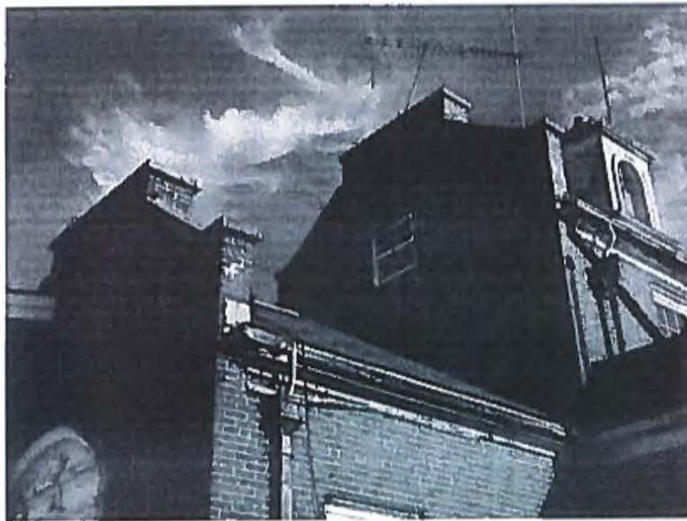
(2.) 1934 Lower & Upper Stepped-Brick Gables (South Elevation/Outer-Face)
