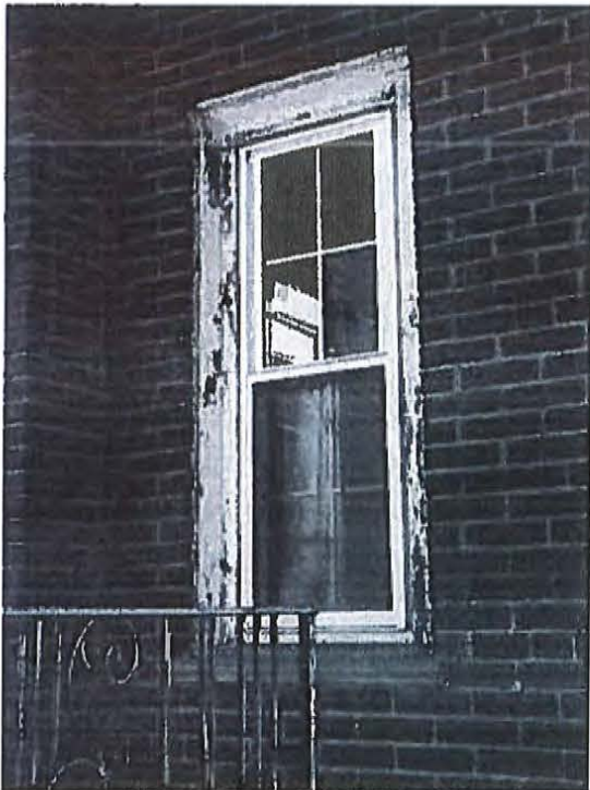
(13.) 1934 Window Surround (South Elevation/South)
