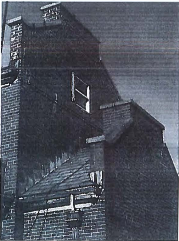
(4.) 1934 Lower & Upper Stepped-Brick Gables (North Elevation/Outer-Face)
