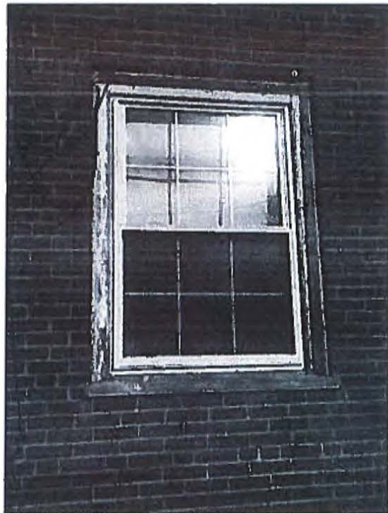
(14.) 1934 Window Surround (East Elevation/South)
