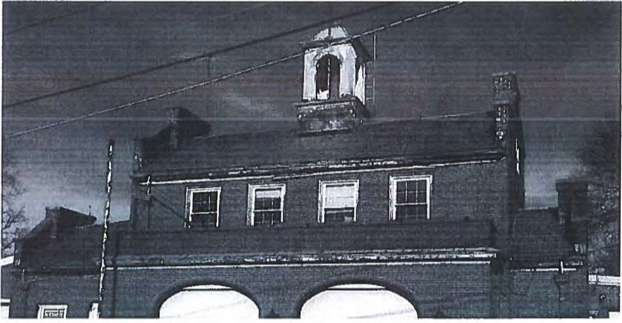
(6.) 1934 Slate Roof – Upper & Lower (East Elevation/Portion Visible from Washington Street)
