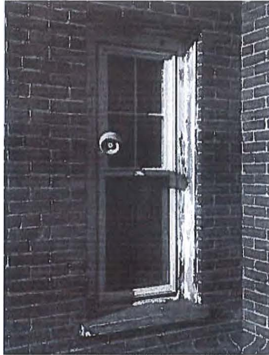
(12.) 1934 Window Surround (North Elevation/North)
