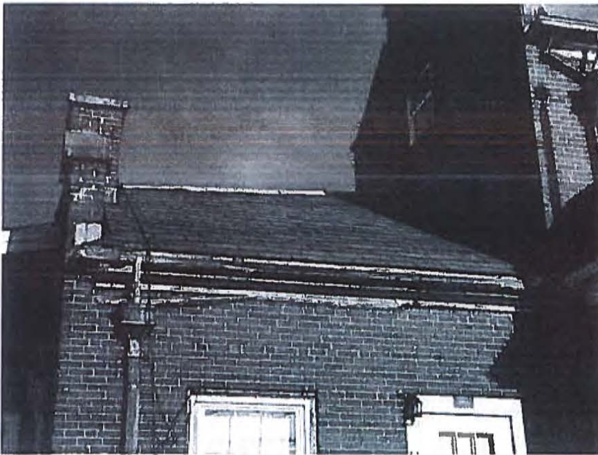
(8.) 1934 Slate Roof – Lower (South-Side/East Elevation/Portion Visible from Washington Street)
