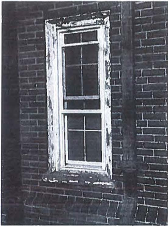
(11.) 1934 Window Surround (East Elevation/North)
