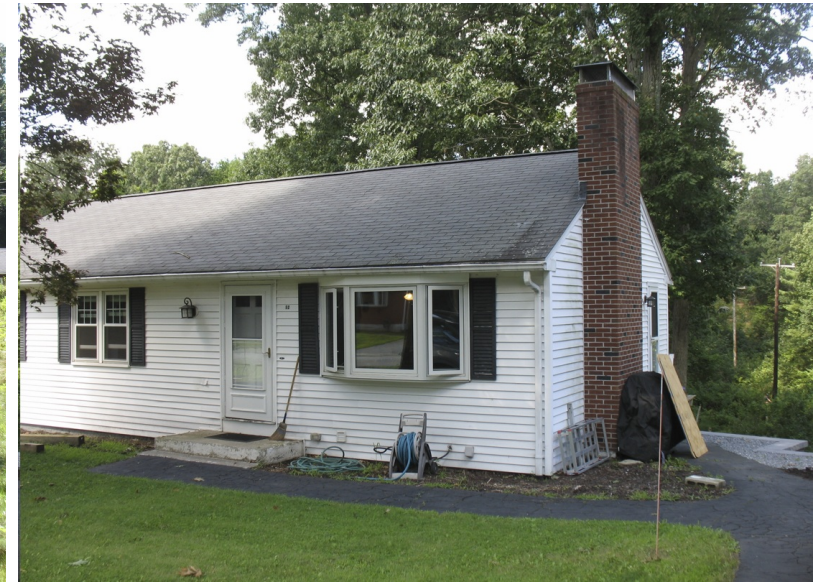
EXISTING CONDITIONS PHOTOGRAPHS Scale: 3/16" = 1'-0"
