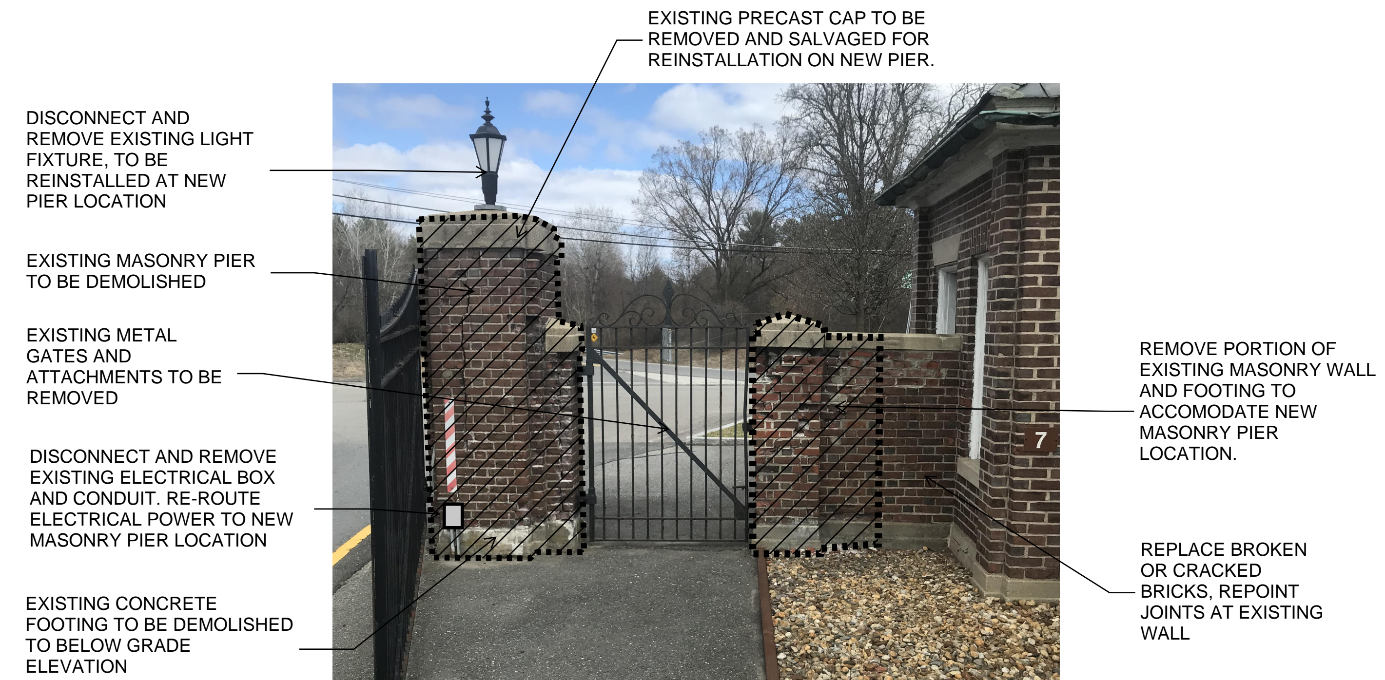
3 PIER C - DEMOLITION
