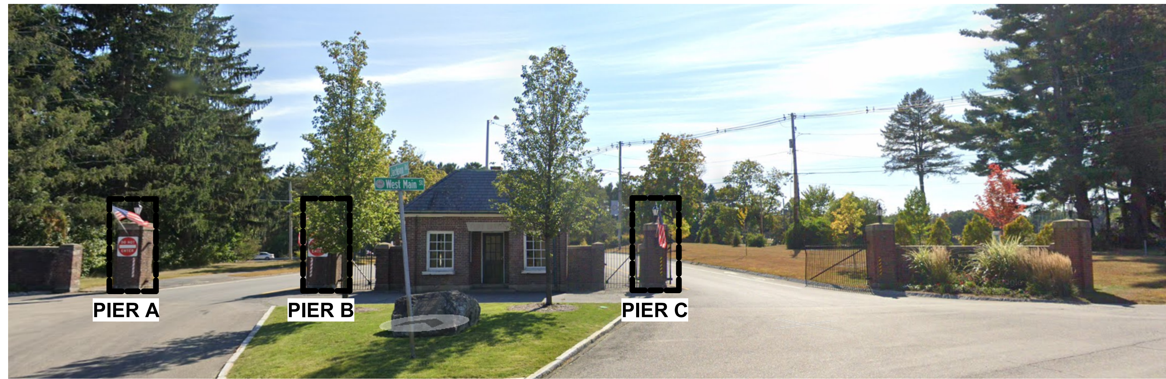
2 PHOTOGRAPHIC ELEVATION - EXISTING CONDITIONS (WEST MAIN STREET)
