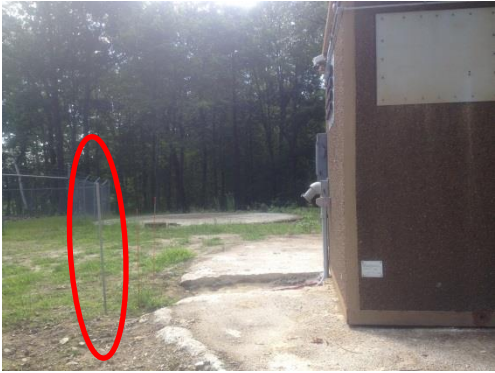
Location of 8' utility ground rods to concrete communications shelter
