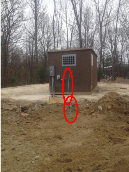
Location of 8' utility ground rods to concrete communications shelter
