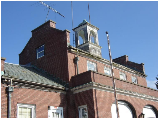
Distinctive "Colonial-Revival" architecture with "stepped-gable ends" and original slate roof.
