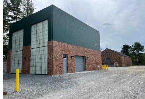
Spectacle Pond Treatment Plant:
