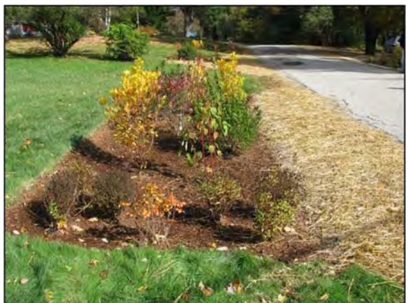
Newly planted rain garden with shrub planting scheme (Mirror Lake watershed, Tuftonboro, NH).
