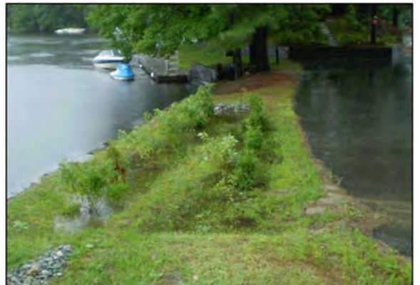
Lakeside rain garden providing storage during a rain storm (Lake Shirley, Lunenburg, MA).
