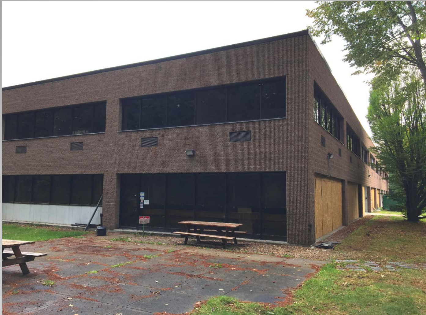
Former Cains Property
