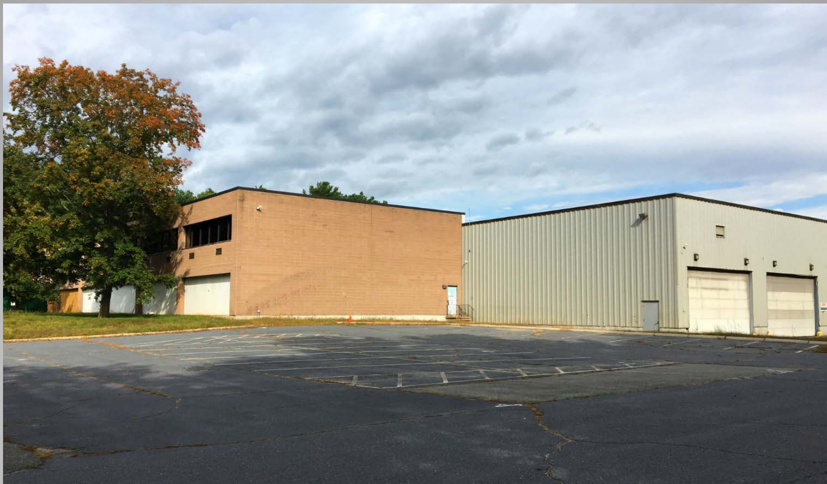
Former Cains Property
