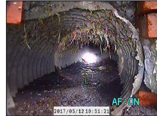
Figure 3-7 Example of a RCP in Excellent Condition (Left) and CMP in Poor Condition (Right)
