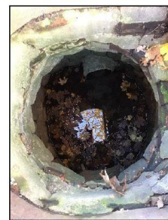
Figure 3-5 Example of a Precast Drain Manhole (Left) and Brick/Block Catch Basin (Right)
