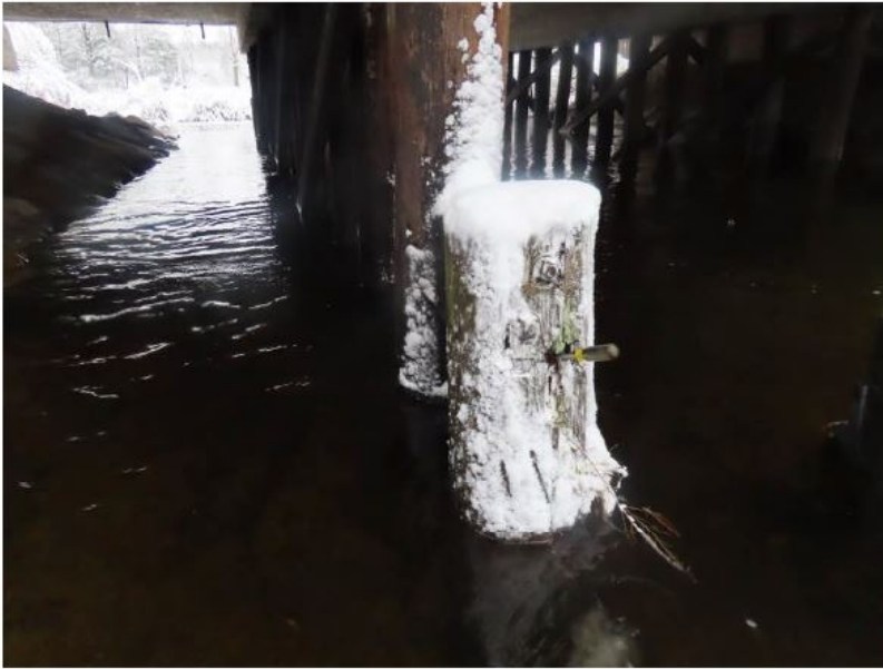
Photo 24: Rot to the battered brace pile at the North end of bent #2.
