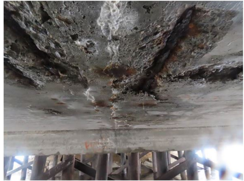
Photo 6: Spall to the center longitudinal joint in span #1 looking East.
