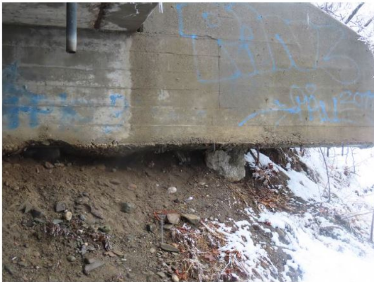
Photo 22: Severe undermining of the East breastwall/wingwall exposing the pile.
