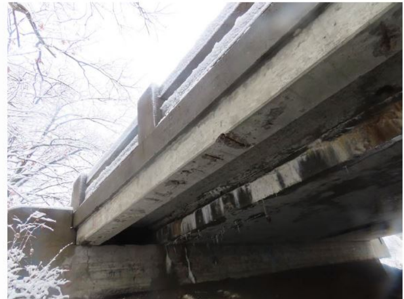
Photo 19: Spalls to the underside of the North sidewalk beam in span #3.
